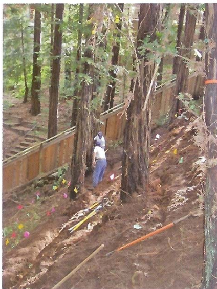
A steep slope installation in California — 65% slope.
