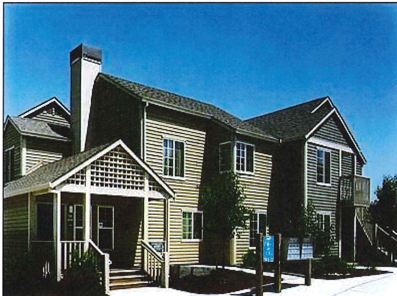
Edgewater Place Apartments - Larkspur, California Sponsor: EAH Housing
