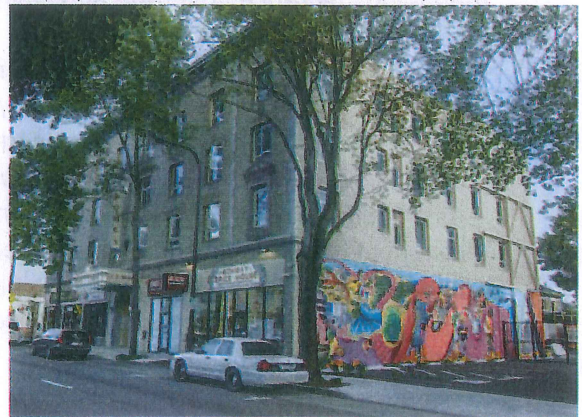
Built in the 1920's, UA Homes was recently rehabilitated and restructured for long-term operating success
