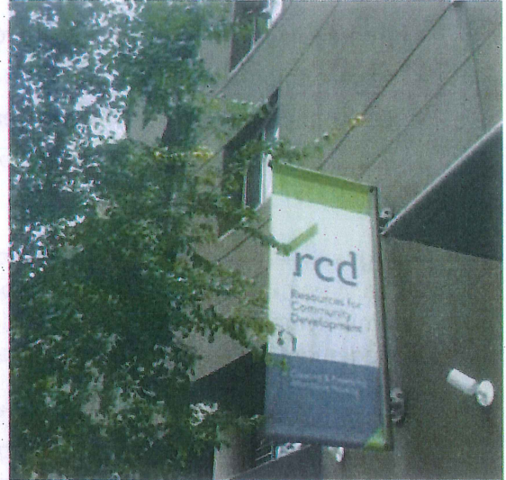
Three commercial spaces, including RCD's headquarters, form the street level retail at Oxford Plaza
