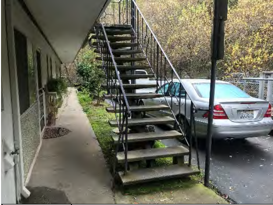
#13 EXTERIOR STAIRS - FRONT
