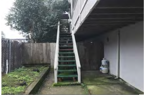
#14 EXTERIOR STAIRS - REAR/FIRE ESCAPE
