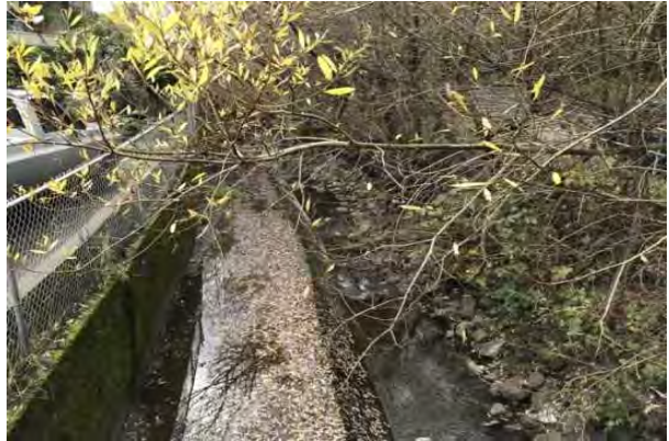
#10 CREEK - FLOOD IMPROVEMENT
