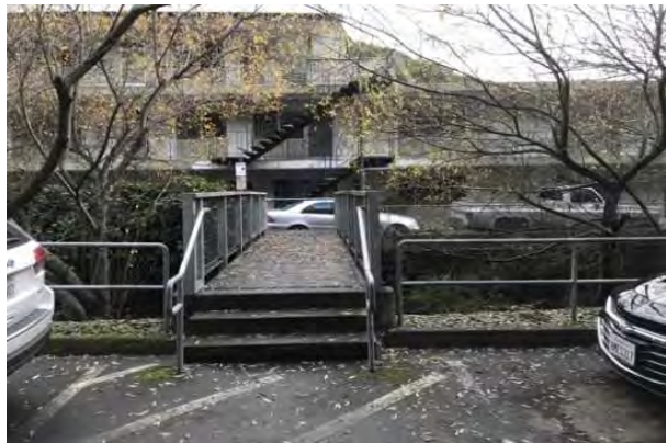
#6 PEDESTRIAN ACCESS BRIDGE
