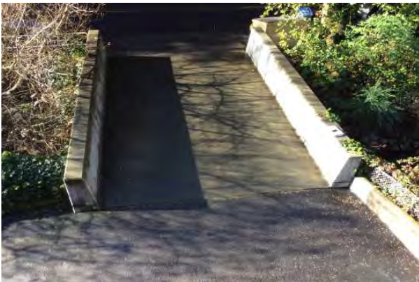
#5 MAIN ACCESS BRIDGE
