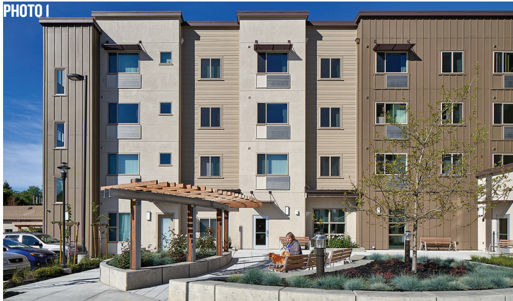
Combination of materials: Stucco, horizontal siding, vertical board & batten
