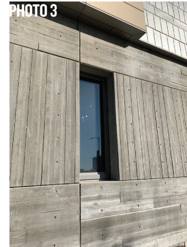
Board form concrete
