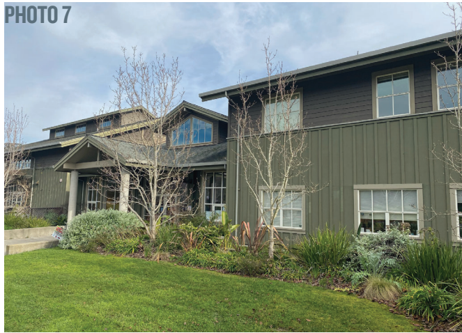
Horizontal Siding over Board & Batten
