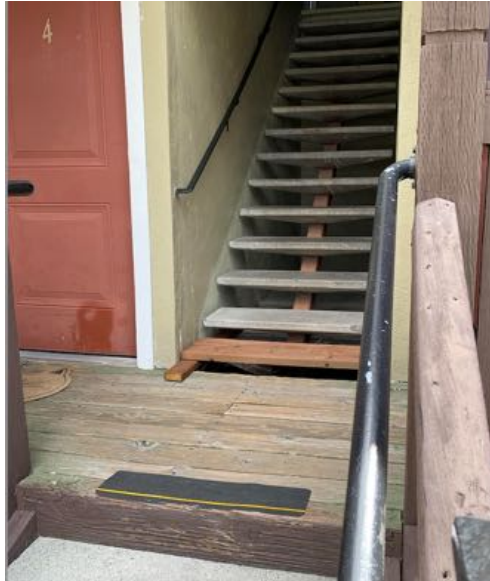
Repair bottom stair tread, add riser closers
