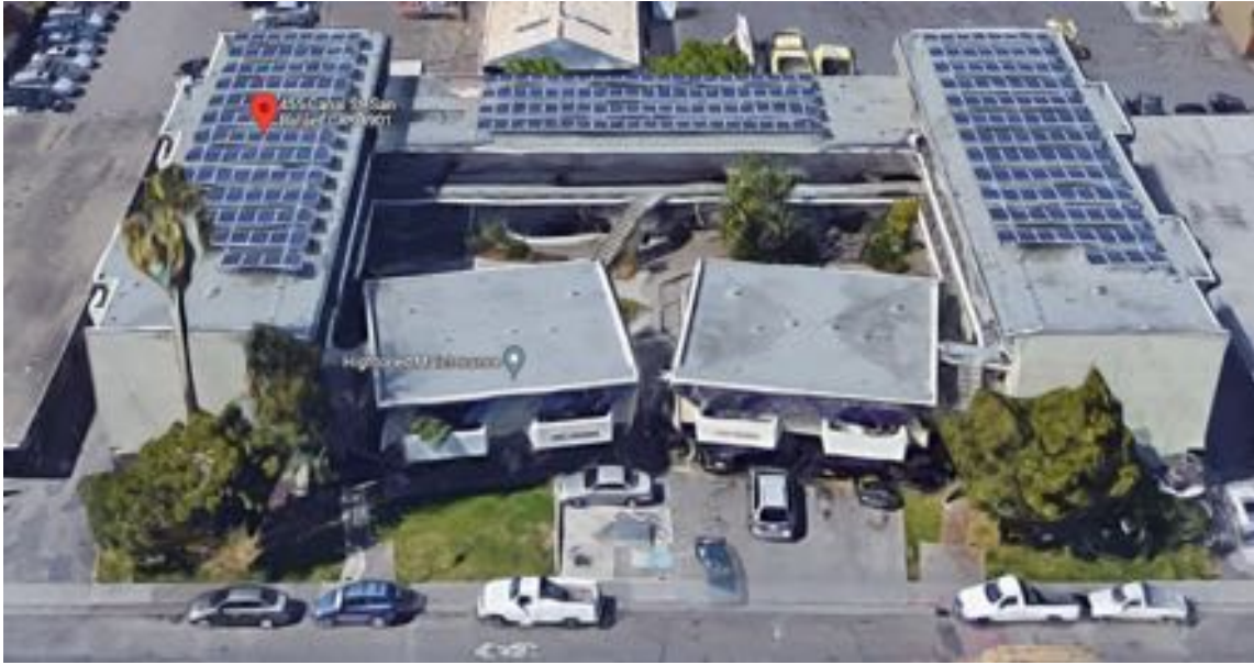
Aerial view – two front 2-story buildings, larger U-shaped building sides and rear.
