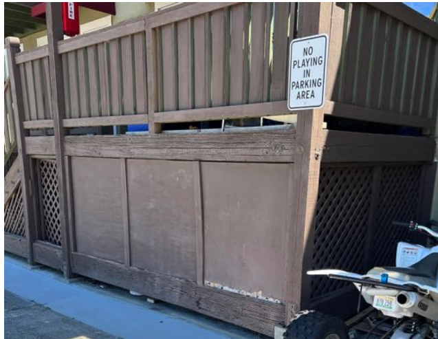
Ground floor entry deck siding
