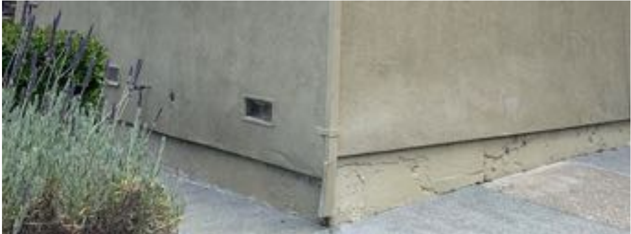
Building base – footing wall – with crawl space vents
