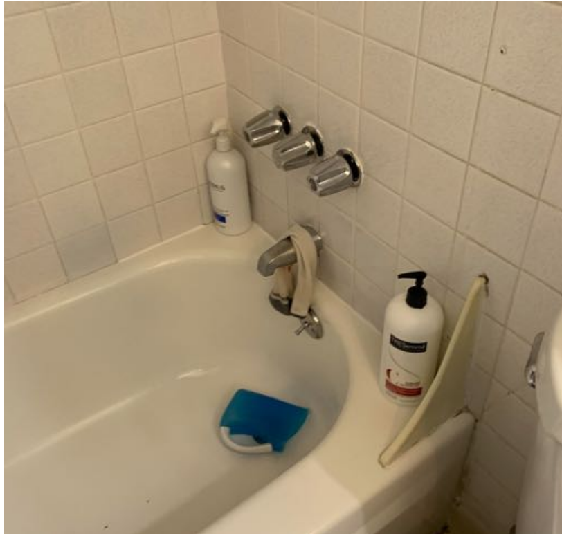
Tub, surround and shower controls
