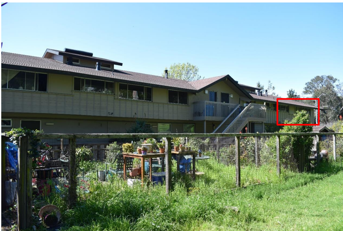
Figure 7: Photograph of low-rise building B-12, rear (east) façade, with approximate location of unit 115 outlined in red, facing northwest. Source: ICF, 4/10/2019.
