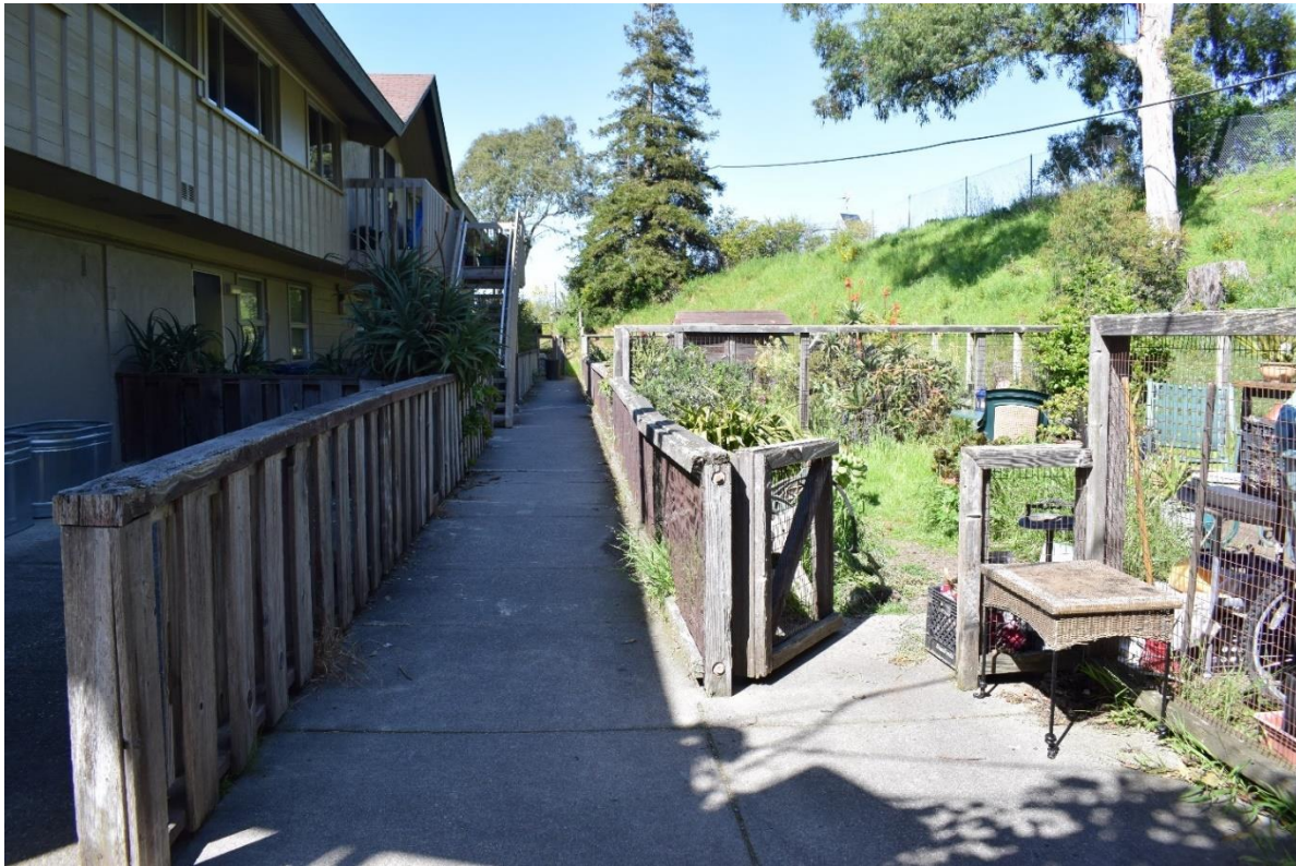
Figure 8: Photograph of low-rise building B-12, rear (east) façade to the left and sloped landscape to the right, facing north. Source: ICF, 4/10/2019.
