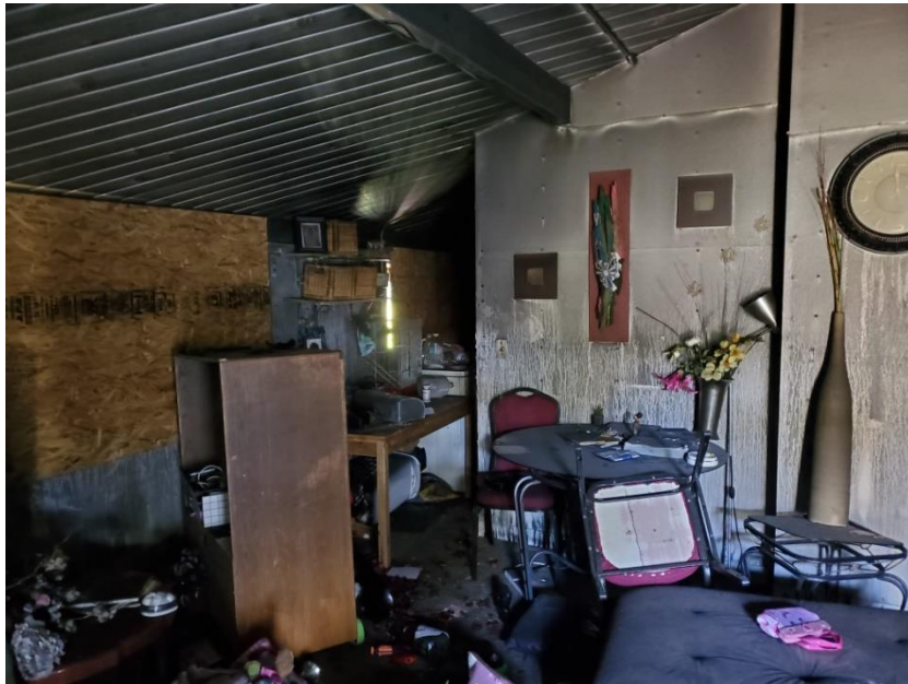
Figure 9: Photograph of interior of unit 115, with smoke damage at the windows, building walls, and roof. Source: MHA, received by ICF on 5/19/2020.
