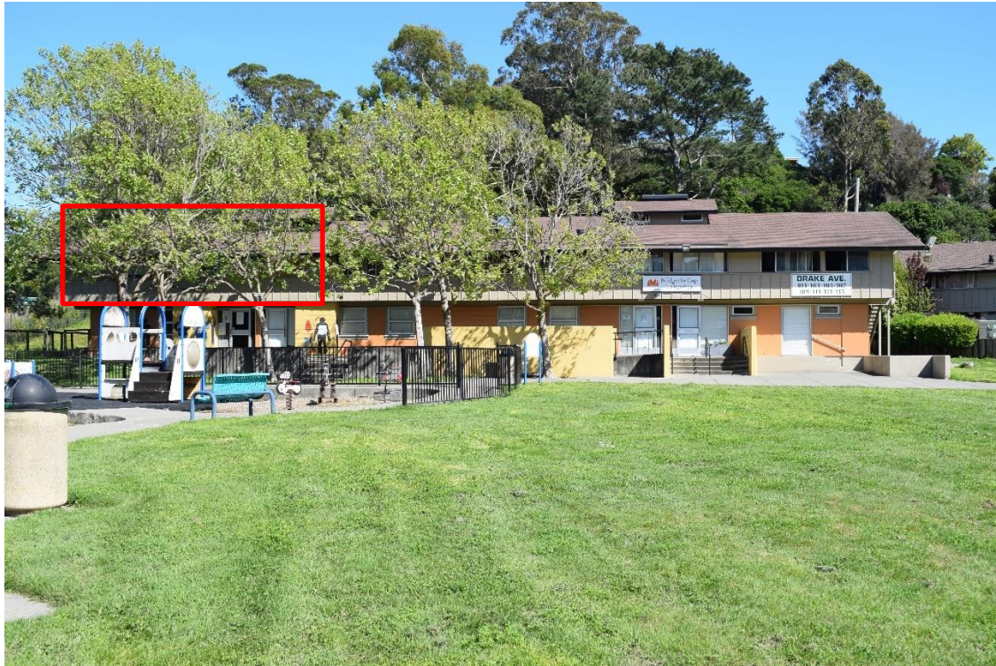
Figure 6: Photograph of low-rise building B-12, primary (west) façade, with approximate location of unit 115 outlined in red, facing east. Source: ICF, 4/10/2019.
