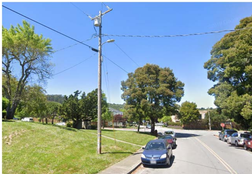
Figure 8. Single utility pole light standard, composed of an extension arm on a utility pole, located along Cole Drive, facing northwest. Source: Google, April 2019.
