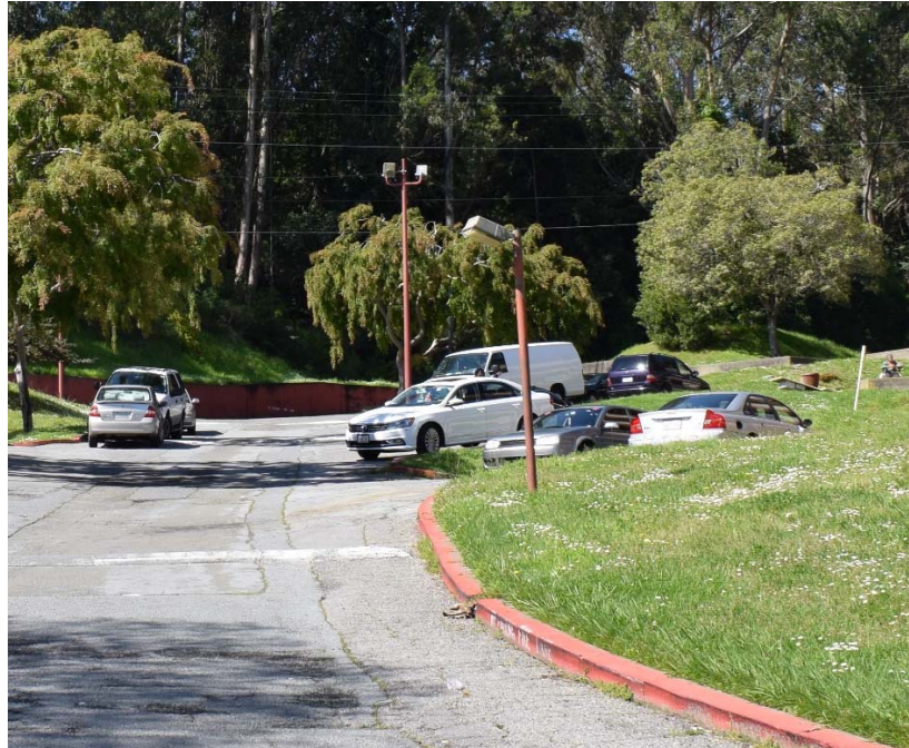
Figure 7. Representative example of a 12-foot Specific Area lighting standard in the foreground. Source: ICF, April 2019.
