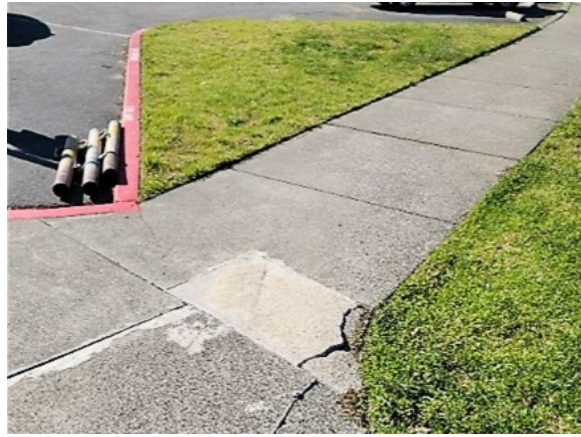
Photo 3 Existing sidewalk along the proposed trenching route, looking southwest. Source: MHA, 2023.
