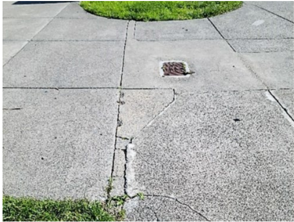
Photo 2 Existing sidewalk along the proposed trenching route, looking east. Source: MHA, 2023.
