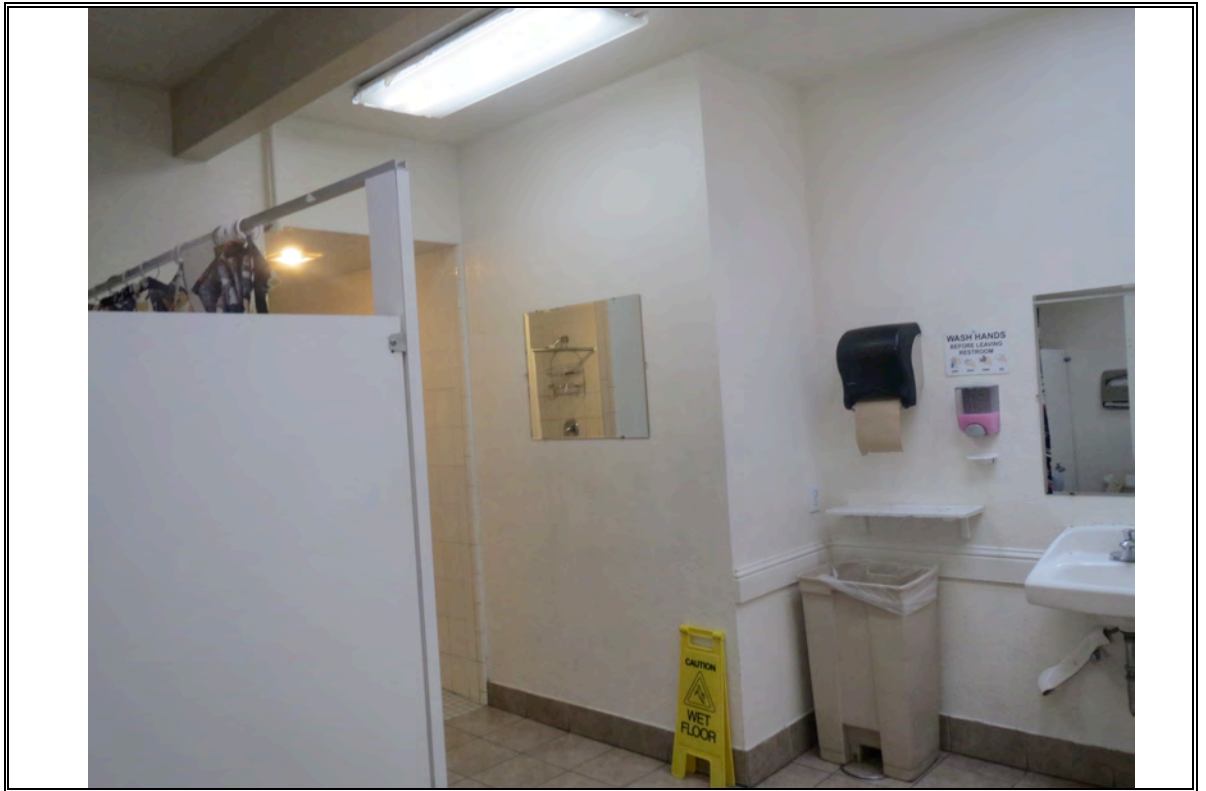
Photograph Number 13: View of the shower area
