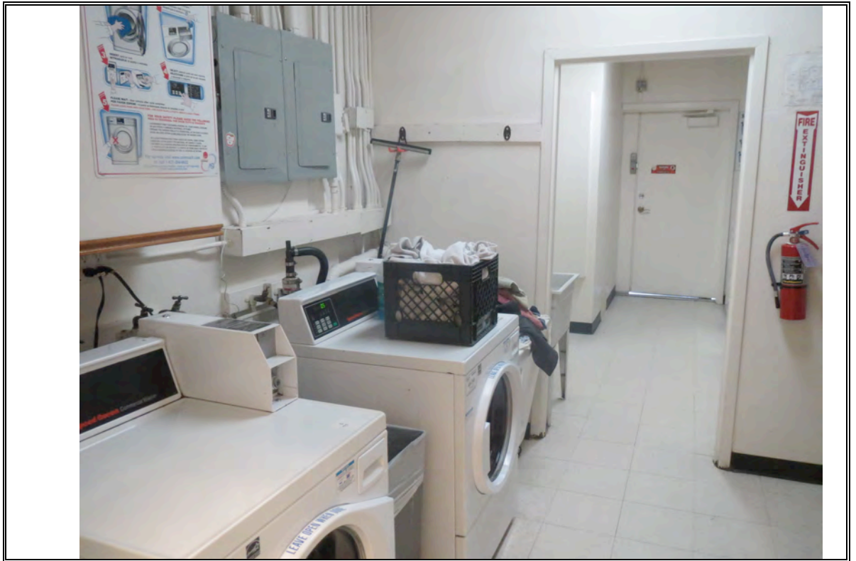
Photograph Number 11: View of the washer and dryers
