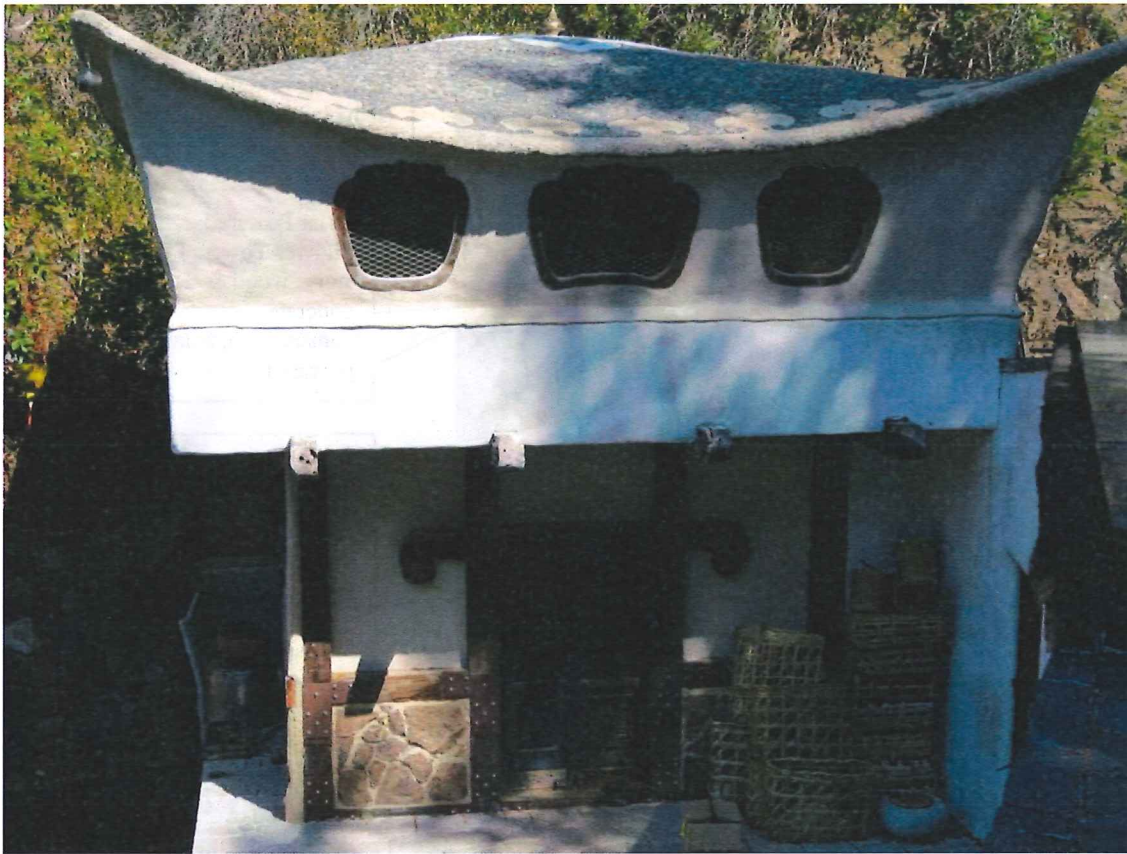
2 stories; first floor is Godown (fortified storage room); concrete & masonry construction; ornamentation: Kathmandu style windows with bird motif on roof.
