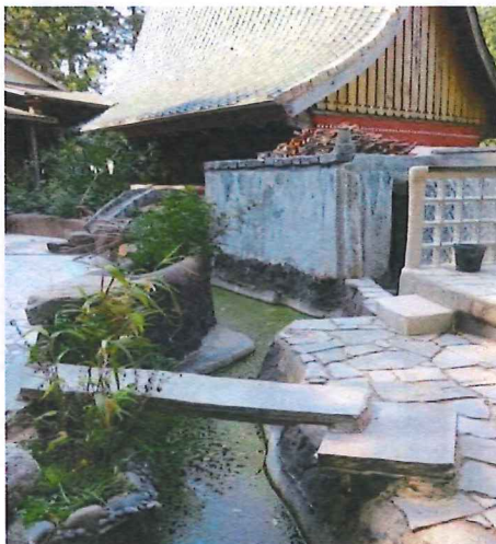
Teahouse (looking from west)
