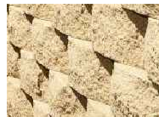
9 KEYSTONE BLOCK RETAINING WALL, COLOR: "BUFF"
