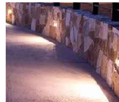
13 EXTERIOR LIGHT FIXTURE AT RETAINING & STAIR WALL, BEGA RECESSED WALL LIGHT WITH SLOTTED FACEPLATE, 5.6 WATT LED COLOR: "BRONZE"
