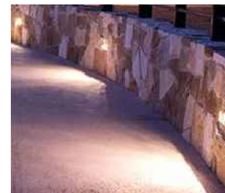
13 EXTERIOR LIGHT FIXTURE AT RETAINING & STAIR WALL, BEGA RECESSED WALL LIGHT WITH SLOTTED FACEPLATE, 5.6 WATT LED COLOR: "BRONZE"
