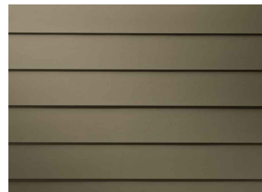
2 HARDIE LAP SIDING, INTEGRAL COLOR: "WOODSTOCK BROWN"
