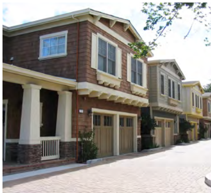
DG-81: Where visible, garage entrances should be recessed and/or accompanied by projecting elements to reduce their prominence.
