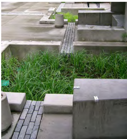
DG-41: One LID strategy involves the incorporation of bio-retention planter boxes as landscape elements.
