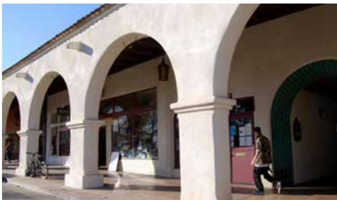
Example of a Gallery with shopfronts
