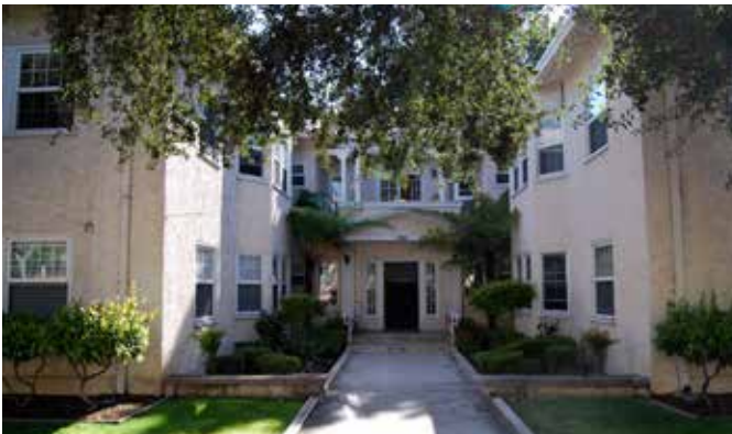
Example of Forecourt
